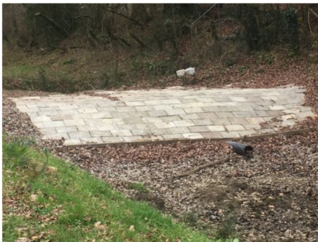
The dam crest cladding.
