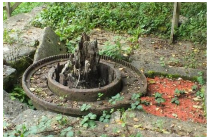
The crane base and rotating mechanism
